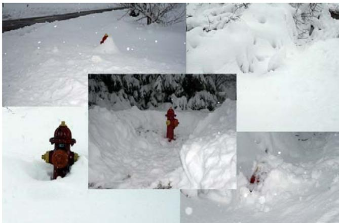
At any given time in the winter, Sun Peaks can receive over 25 centimeters (10 inches) of snow within a 24 hour period. This snow along with the plow trucks can partially or completely covered hydrants at Sun Peaks. This can make it very hard to locate and use these hydrants in an emergency. It only takes 75 centimeters (30 inches) to completely cover most fire hydrants if not attended to.
